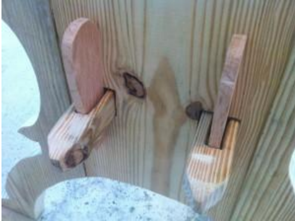
Assembled legs with tenons firmly wedged in mortises
