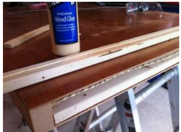
Plug the open end of your hollow door with strips of wood and glue
